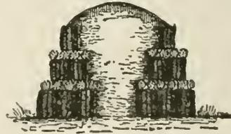
rectangular space of about 15 feet in width from out to out, and about 24 feet in length, perpendicular to the parapet. A second row is placed within this and touching it, and a third row inside of the second. The area thus inclosed is filled in with earth to a level with the top of the gabions. Six rows of large fascines are next laid on the gabions to support a second
